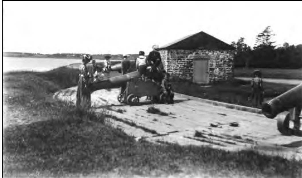
Figure 4.2- 13: Photograph of Fort Edward circa 1900. Note the wooden platform and stone magazine. 46
