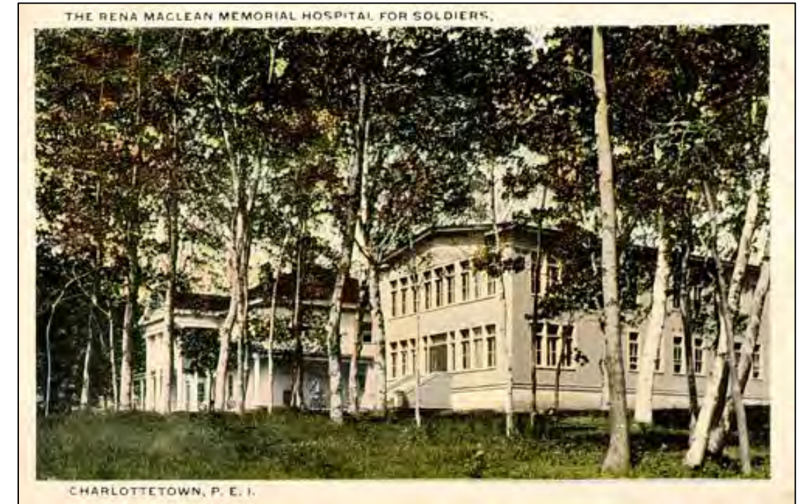
Figure 4.2- 15: Undated postcard showing the Rena McLean Memorial Hospital in relation to the Government House. 50
